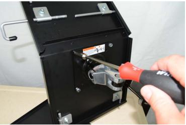
\* Installation tip – tilt the VESA plate so that the hinged door doesn't fall on fingers during installation
